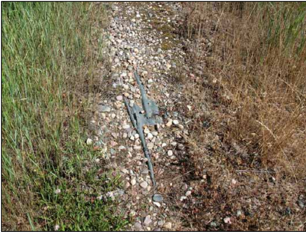
Photograph P35. Photograph depicting a portion of exposed pond liner at Pond 6 (July 2015).
