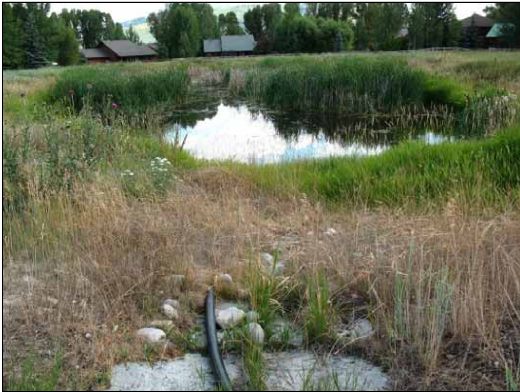
Photograph P40. Photograph depicting the northern portion of Pond 7, concrete inlet structure, and supplemental water supply pipe, looking south (July 2015).
