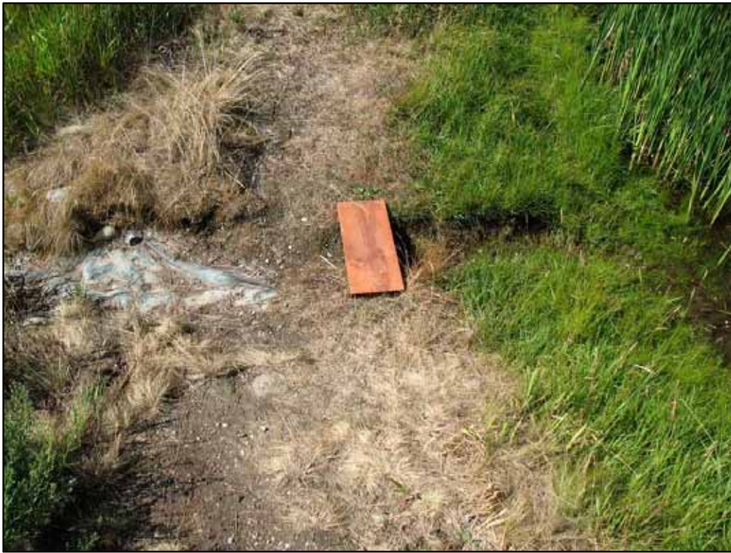
Photograph P5. Photograph depicting the outlet of Pond 1 and a portion of exposed liner.
